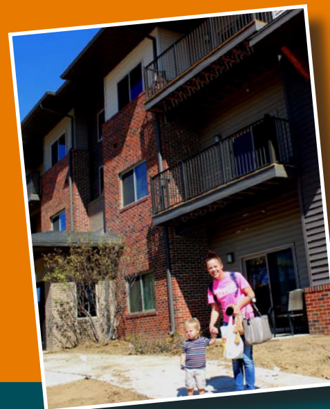
New construction is popping up all over the community, including The Summit at Sunnybrook Village on Sioux City's east side.
